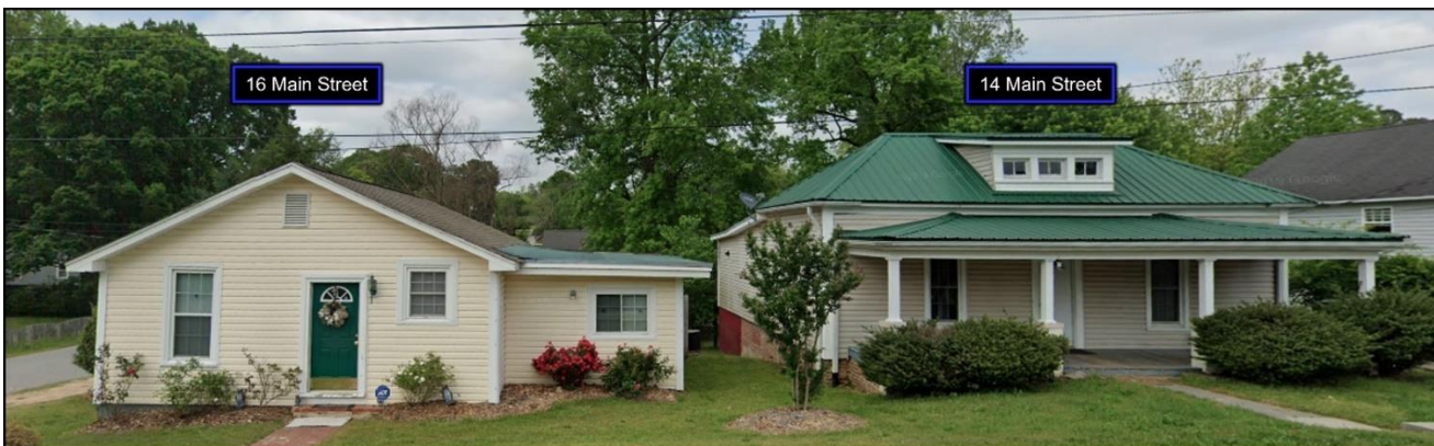
Google Street View – Structure Separation
