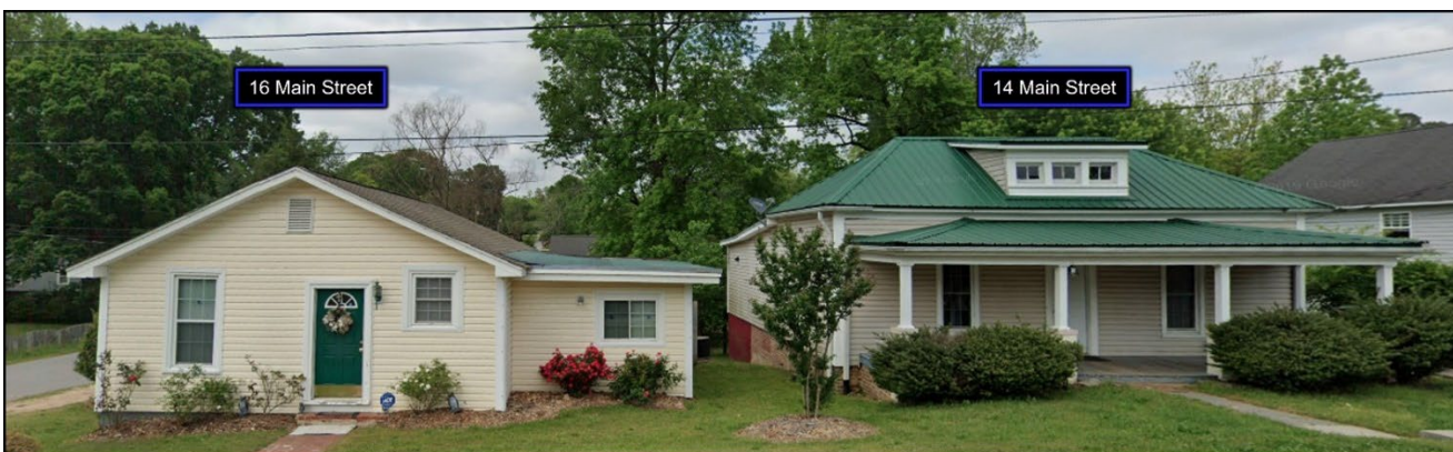
Google Street View – Structure Separation
