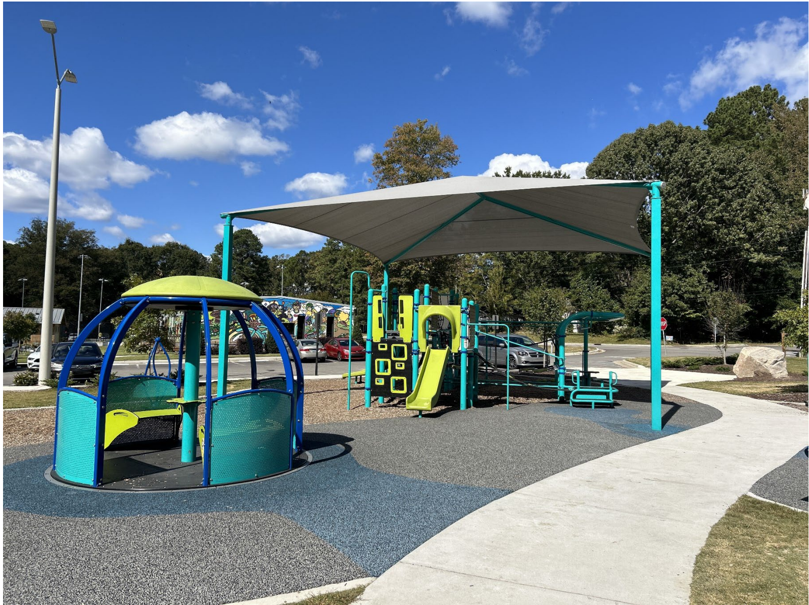
Harper Park Shade Structure
